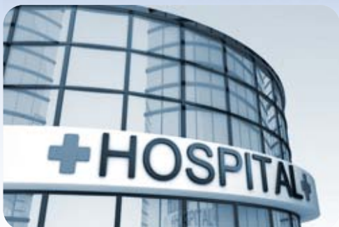
HOSPITAL WASTE WATER
