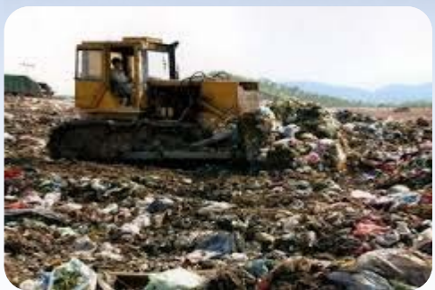
SOLID WASTE ODOR CONTROL
